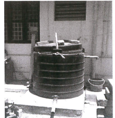
Kitchen waste Biogas Plant
