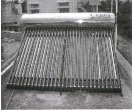
Evacuated Solar Water heater
